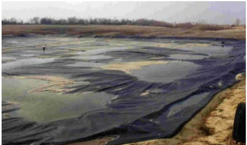
Outputs and Uses. Recent biogas production levels are unknown because the gas meter broke and was not yet replaced. However, in mid-summer 1998, the digester was producing 36,000 cfd (prior to all-in all-out management). The biogas is used to run a Burnham boiler (pictured below) that serves the sole purpose of heating the digester. Excess biogas is flared. Digestate is land spread on croplands with a corn and soybean rotation.
