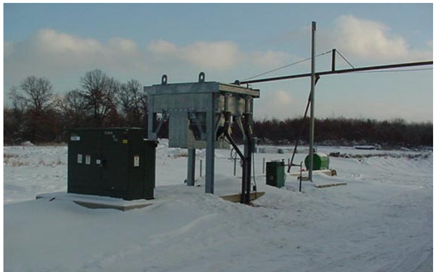
Photo: Alliant Energy, Inc.
