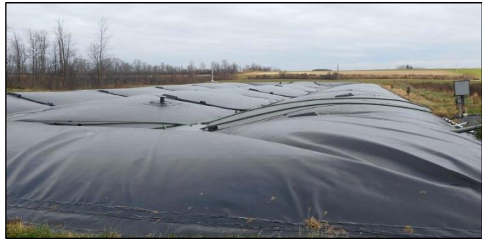
Spruce Haven Farm anaerobic digester.
