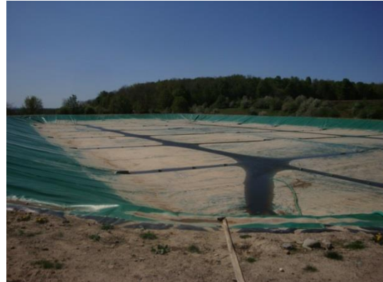
Covered Manure Storage at Fessenden Dairy
