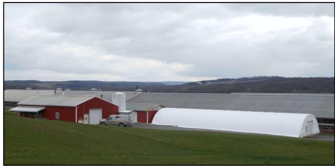
Twin Birch Farm anaerobic digester and biogas utilization building (foreground).
