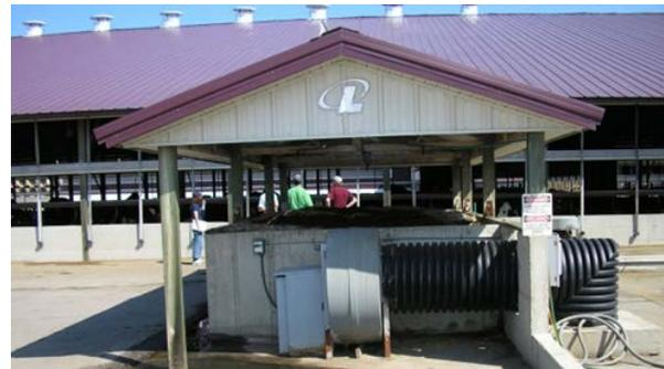
Figure 2. Biofilter treating emissions from a barn manure collection pit at a MN dairy<sup>[3]</sup>.
