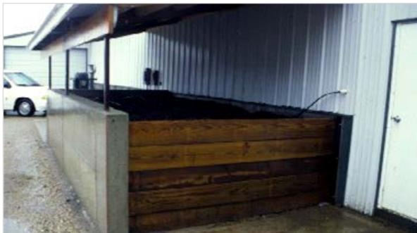
Figure 5. Biofilter treating air from a manure pit inside a SLS building with removable wooden wall for easy media replacement<sup>[3]</sup>.
