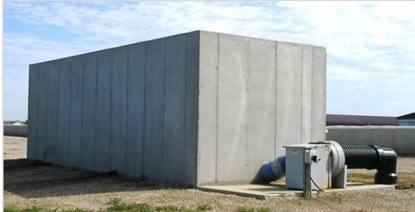
Figure 4. A large 6 ft. deep biofilter at a dairy in MN was designed to treat contaminated air from both an anaerobic digester effluent and the SLS building<sup>[3]</sup>.
