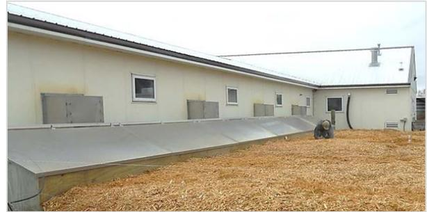
Figure 6. A low-cost, open-bed biofilter treating wall fan exhaust from a swine nursery barn.
