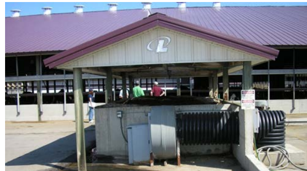
Figure 2. Biofilter treating emissions from a barn manure collection pit at a MN dairy [3] .
