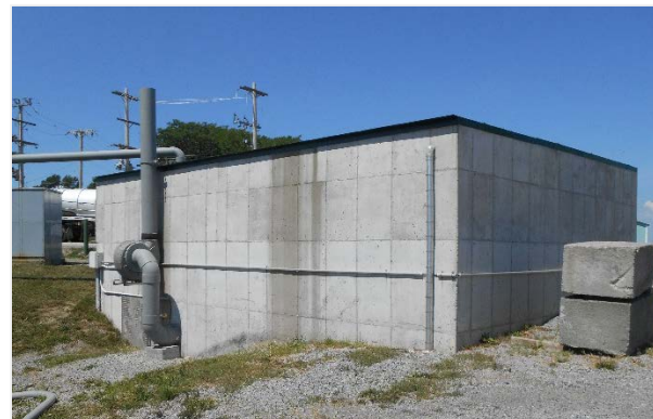
Figure 3. Biofilter at a NY dairy treats odors from manure and food waste reception pits.
