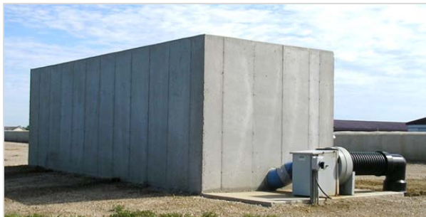
Figure 4. A large 6 ft. deep biofilter at a dairy in MN was designed to treat contaminated air from both an anaerobic digester effluent and the SLS building [3] .
