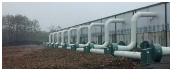
Figure 7. Open-bed biofilters treating exhaust air from a large composting facility [4] .
