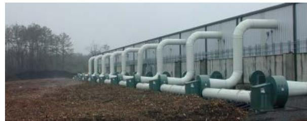
Figure 7. Open-bed biofilters treating exhaust air from a large composting facility<sup>[4]</sup>.
