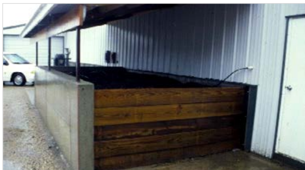
Figure 5. Biofilter treating air from a manure pit inside a SLS building with removable wooden wall for easy media replacement [3] .
