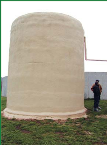
Farber Farms Fixed film vertical digester.
