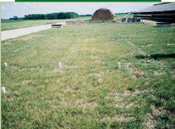
Noblehurst Hard-top plug-flow digester.
