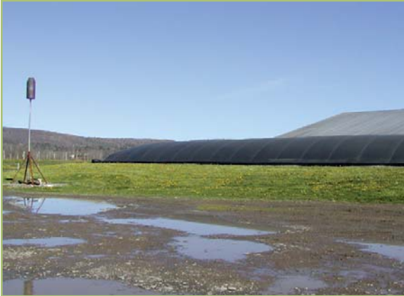
AA Dairy Soft-top plug-flow digester.
