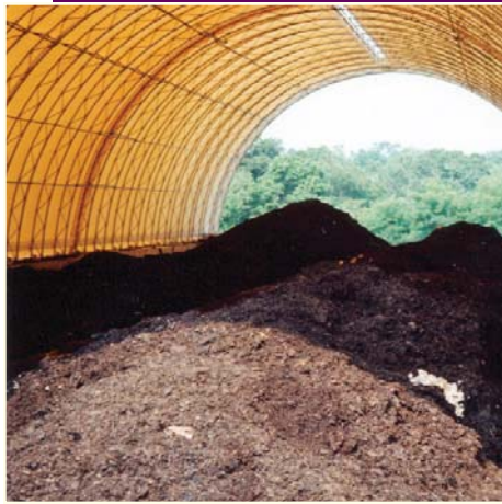
Newly built Coverall building for all-season composting.
