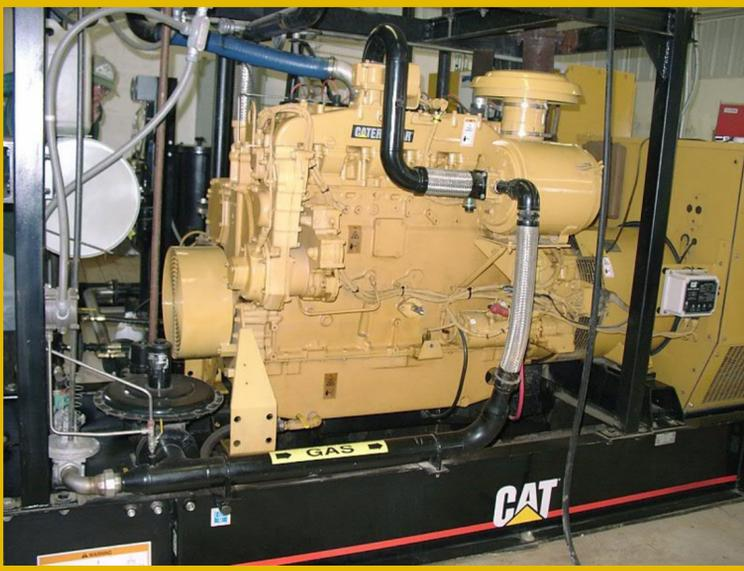
Engine generator running on biogas
