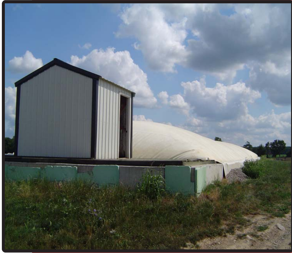
Digester and influent pit building
