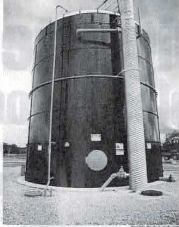
AN IFAS FIXED-FILM anaerobic digester cuts odor by 90% or more at the University of Florida Dairy Research Unit.
