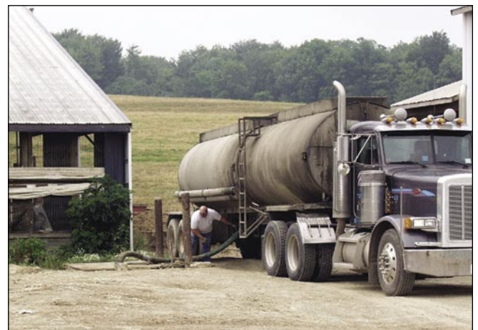
Food waste being pumped into the reception pit of an anaerobic digester at Matlink Dairy Farm, Clymer, Chautauqua County, N.Y.
